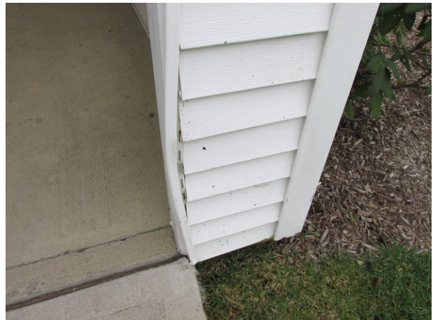
Siding damage
