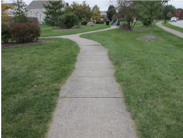
Concrete sidewalk overview
