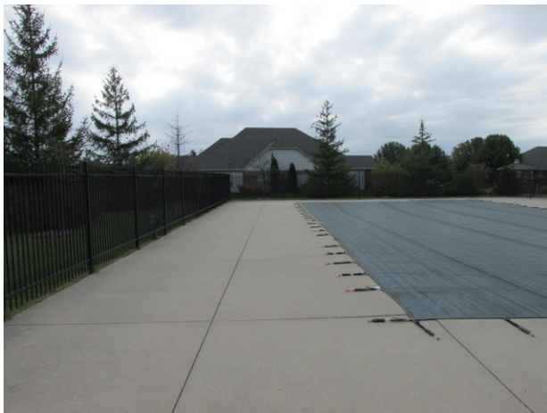
Concrete deck at pool
