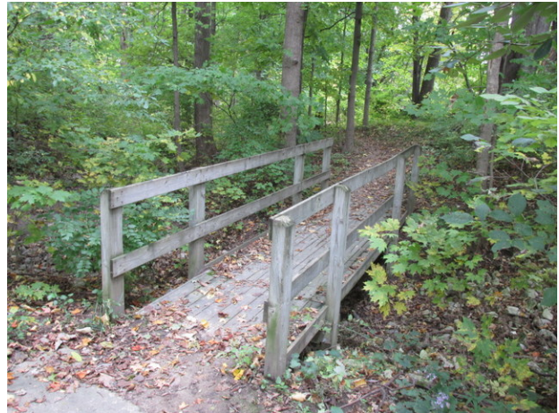
Pedestrian bridge along one of the rustic trails
