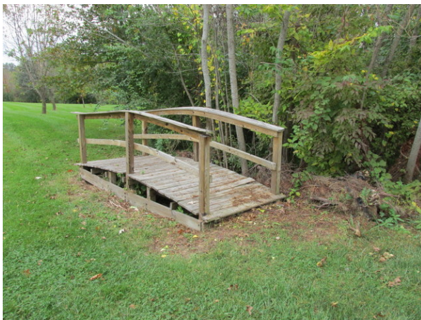
Pedestrian bridge near playground on Split Rock Way
