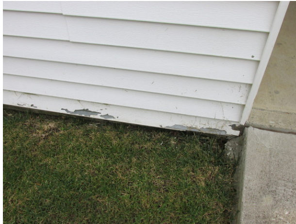
Siding damage
